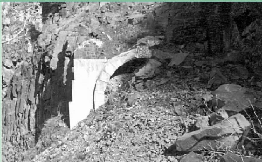
The west end of Twin Tunnels prior to excavation.
