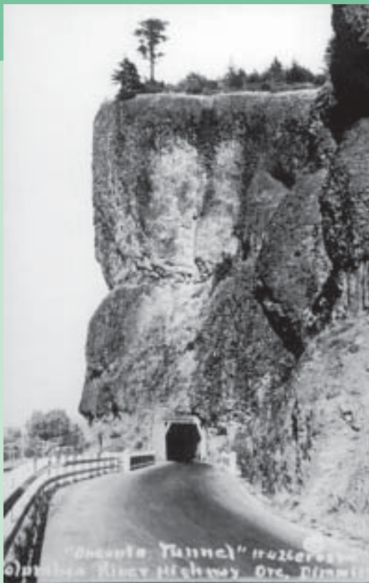
Oneonta Tunnel was the next point of interest east of Multnomah Falls on the old Columbia River Highway.
