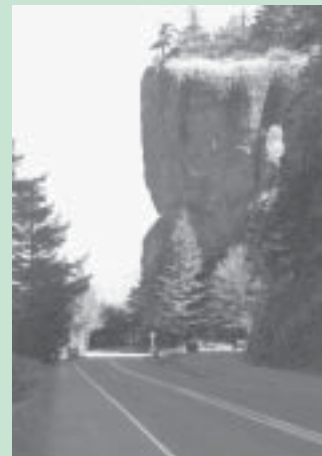
The Historic Highway is currently re-routed around the rock bluff where Oneonta Tunnel was located.
